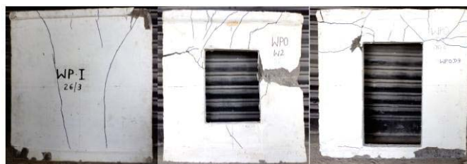
Fig. 12 Crack Patterns of UHPC wall panels
